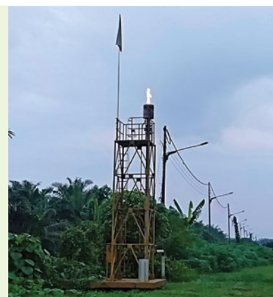
Biogas Flare Stack
